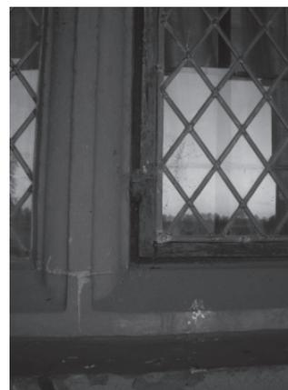
Mullion detail: 150mm thick containing panes of between 800mm and 1400mm tall
