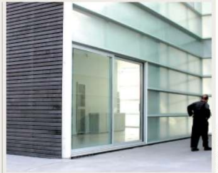
The facade appears as a series of thin metal shelves supporting the glazing.
